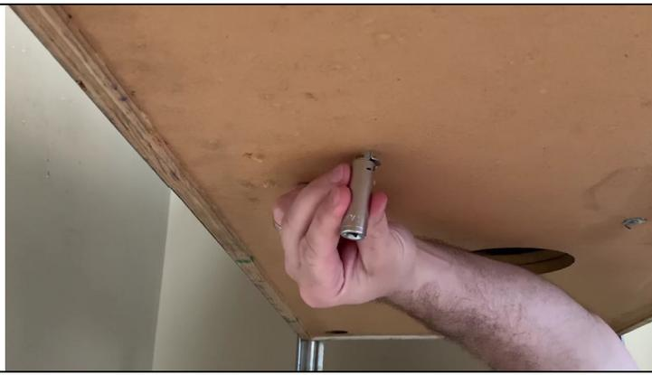
**Step 6:** Once you get all 4 screws drilled, go underneath and hammer in the 4 tee nuts. Sys 7 & 9 installations will use the included washers and locknuts instead. Use the 1/2" deep socket to help so you don't smash your fingers. Hammer the tee nuts as far in the cabinet as they will go. If they do not go all the way in they will finish flush when you screw in the hex screws in the next step.
