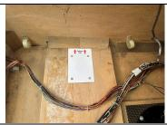
Step 7b: Shaker Motor Installation Included is a custom drill guide with 4 pre-drilled holes that you will use to drill the 17/64" holes in the cabinet. Place the drill guide against the side wall in the spot you believe you want the motor to be mounted.
