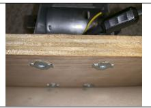
Here is an example of properly installed tee nuts. See how they rest flush with the wood. If your tee nut falls out while you are trying to screw them in, that means you probably did not hammer them in far enough. Make sure you take a pair of pliers and straighten out the prongs before you try to re-install it.
