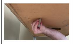
Step 7e: Shaker Motor Installation Once you get all 4 screws drilled, go underneath and hammer in the 4 tee nuts. Use a 1/2" deep socket to help so you don't smash your fingers. Hammer the tee nuts as far in the cabinet as they will go. If they do not go all the way in they will finish flush when you screw in the hex screws in the next step.
