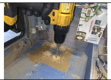
Step 6d: Shaker Motor Installation
